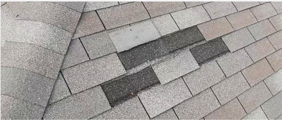
MISSING SHINGLES
